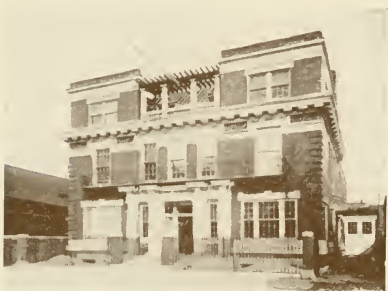
RELIEF STATION OF BOSTON CITY HOSPITAL
